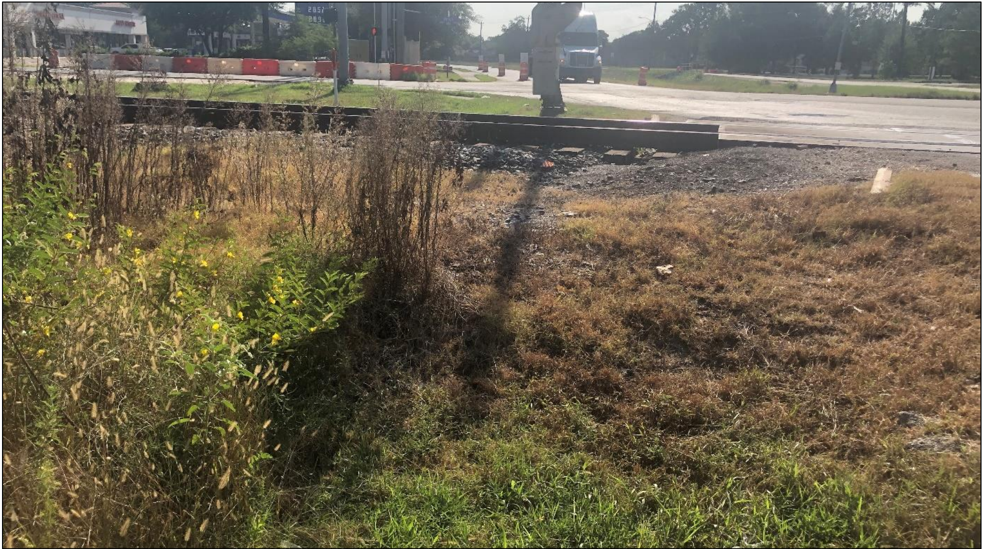
Figure 21. The Union Pacific railroad at the intersection of Little York Rd. and Hirsch Rd.
