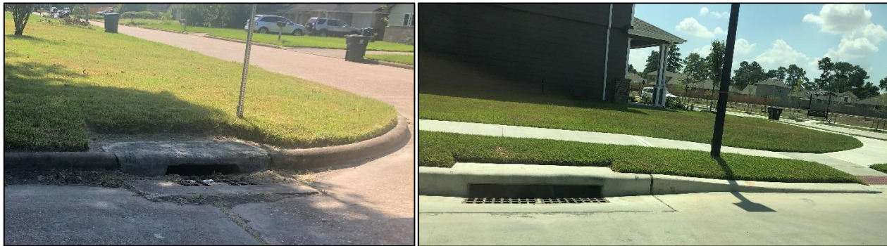
Figure 20. On the left, a drainage inlet in the old section of Northwood Manor. On the right, a drainage inlet in a newly developed neighborhood of Northwood Manor. Pictures by Camille Chenevert.
