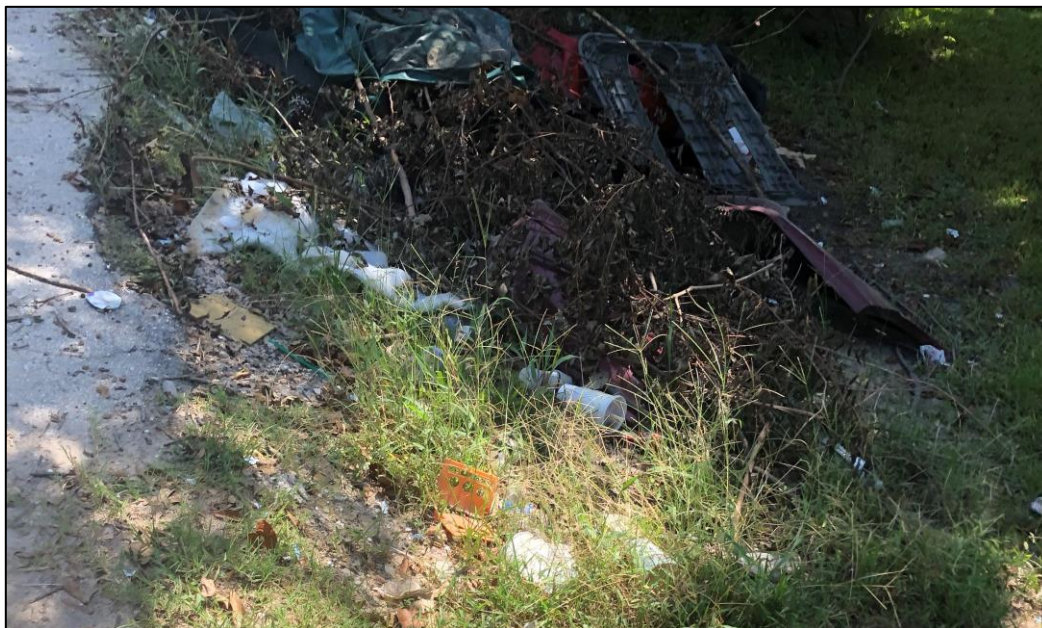
Figure 16. Open drainage ditch in Northwood Manor with trash piling up and obstructing drainage. Picture by Camille Chenevert.
