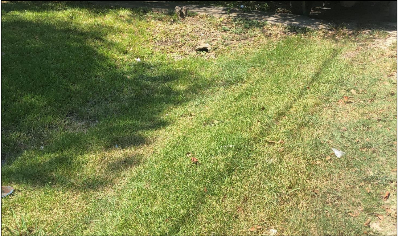
Figure 13. Picture of open drainage ditch in Northeast Houston with culvert non-functional. Photo by Camille Chenevert.
