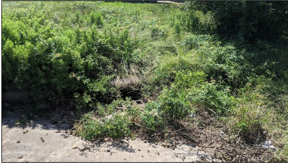
Figure 19. A drainage inlet on an uninhabited property in Northwood Manor which is almost completely covered by overgrown plants and debris. Picture by Sarah Swackhamer.
